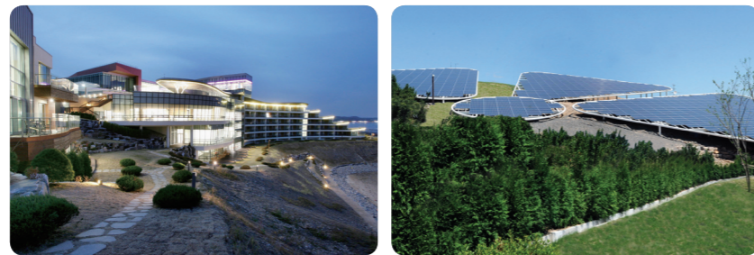
The Homeplus Academy is equipped with solarpowered generation system that reduces 526 tons of CO 2 .
